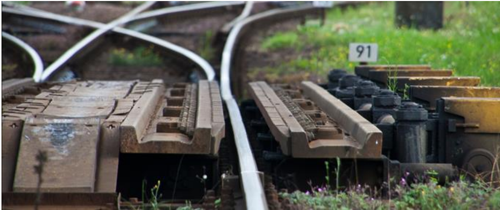
Figure 3: Ramp retarder in München-Nord [Source: jrschmidt-photos.de]
