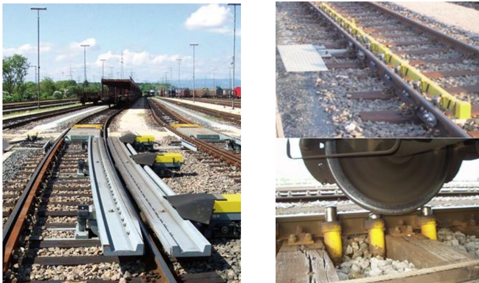
Figure 4: Automatic clasp (beam) retarder (left); Piston retarders in working position (right) [Source: wikipedia.org]
