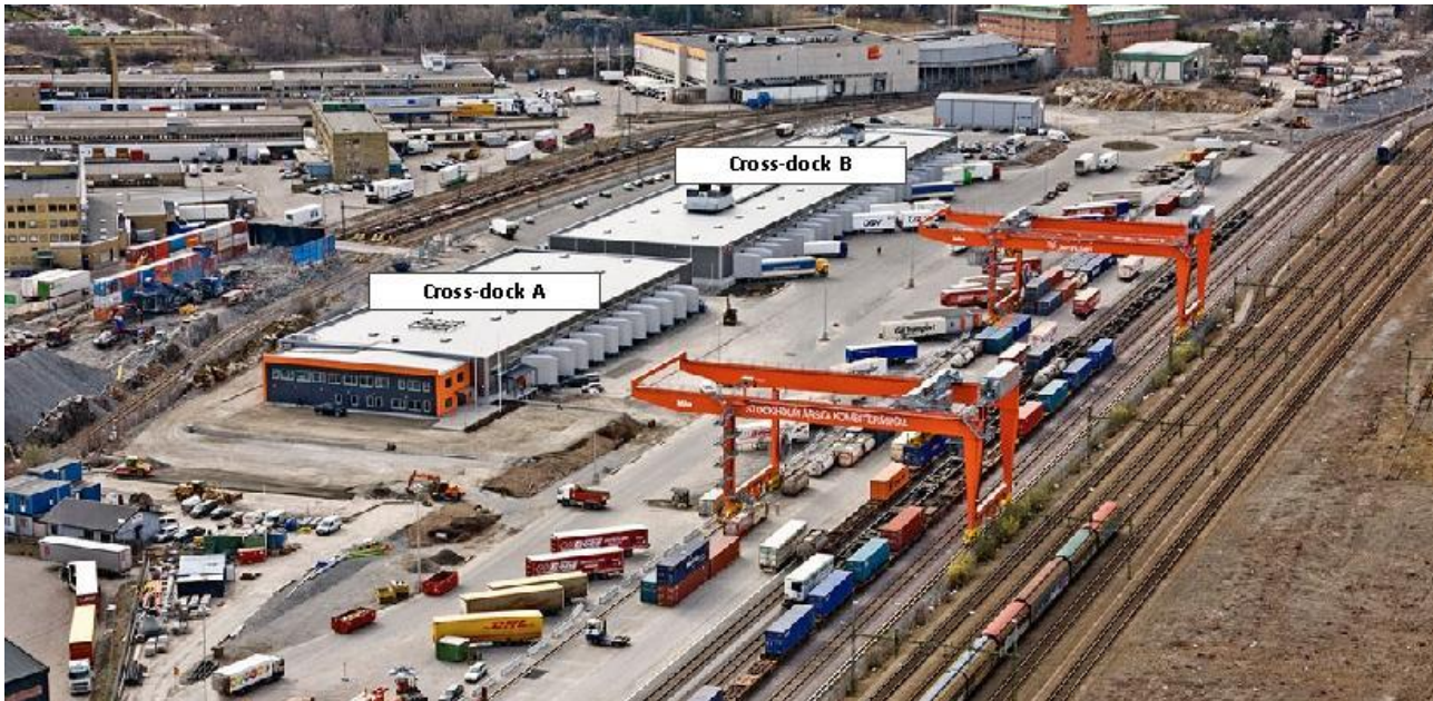
Figure 18: Stockholm Årsta Intermodal Terminal [Source: Jernhusen]
